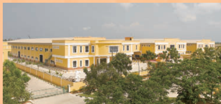
KING'S production facility in Batam
